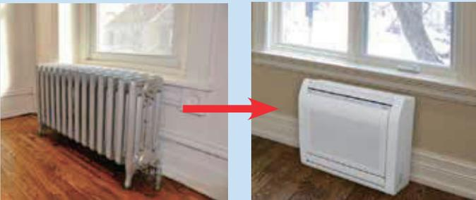
At less than 24" high and 30" wide, floor mount models fit easily under a standard window and can replace a radiator twice its size while producing more capacity.
