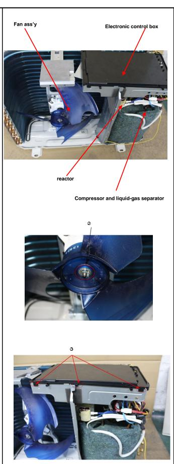
Unfix the hooks and then open the electronic control box cover.
