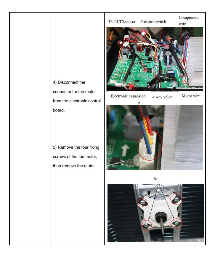
Electrical How to remove the parts electrical parts. 1) After finish work of item 1 and item 2, remove the connector for the compressor 2) Pull out the two blue wires connected with the four way valve. 3) Pull out connectors of the, condenser coil temp. sensor(T3),outdoor ambient temp. sensor(T4) and discharge temp. sensor(T5). 4)Disconnect the pressure switch connector.
