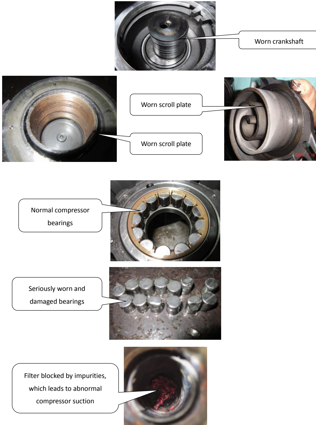
Figure 5-4.17: Effects of spoiled compressor oil
